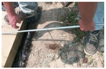
Step 2 - Once you have driven the anchor into the ground, Pull the drive steel out of the ground and insert it into the loop at the end of the cable. Pull cable out of the soil 2 to 3 inches. This will rotate the anchor into a horizontal (locked) position. Now you can mount the anchor to your greenhouse base.
