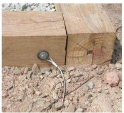
Step 3 - Take the loop at the end of your cable and place a bolt through it so that the cable is between a washer and the greenhouse base. Secure the bolt to the base and you are done. Follow this process for each corner of the greenhouse.
