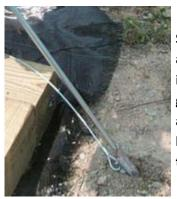
Step 1 - Place the earth anchor in the ground approximately 6 inches away from the corner of your greenhouse base. Put the drive steel inside of the anchor and use your hammer to drive it into the ground. A 3 or 4 lb. hammer will be heavy enough to drive the anchor in most soils. A larger hammer may be needed to penetrate hard soils. Drive the anchor until the end of the cable barely touches the edge of the greenhouse base.
