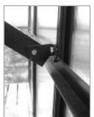
The other end is fastened to the ridge. You can use a self-drilling screw (supplied) or pre-drill the hole using 9/16" drill bit. 3
