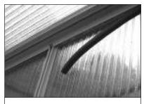
After the polycarbonate panels have been installed, take the round foam and fill the space between the panels and the aluminum
