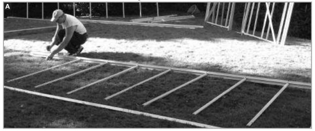
Lay out the sidewall with the gutter at the top-base at the bottom (*See Pic A*). You will notice that each sidewall glass bar has a straight and an angle cut. The straight end fits against the base (*See Pic B*) and the angle goes towards the gutter (*See Pic C*). Always face the bolt slot in the glass bar towards you.
