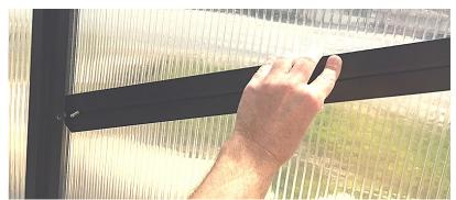
Now that you have all of the bolts in place, insert the support bar behind the inner lips of the greenhouse frame members, and tilt the support bar at an angle. Keep the bottom end of the support bar tight against the greenhouse frame to keep the bolt from sliding out until you reach the pre-drilled hole. Insert the bolt through the hole and secure it with a nut. Now remove the nut from the other side of the support bar and lower it into
